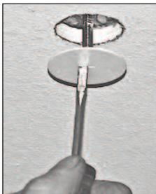
**STEP 4** - Insert the threaded stem of the cover plate into the threaded hole next to the RCA plug. Snug the plate up to the ceiling with a flat blade screw driver. The stem length allows for ceiling panel thickness of 1/2" thru 2"
